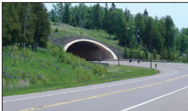
Lafayette Bluff Tunnel
